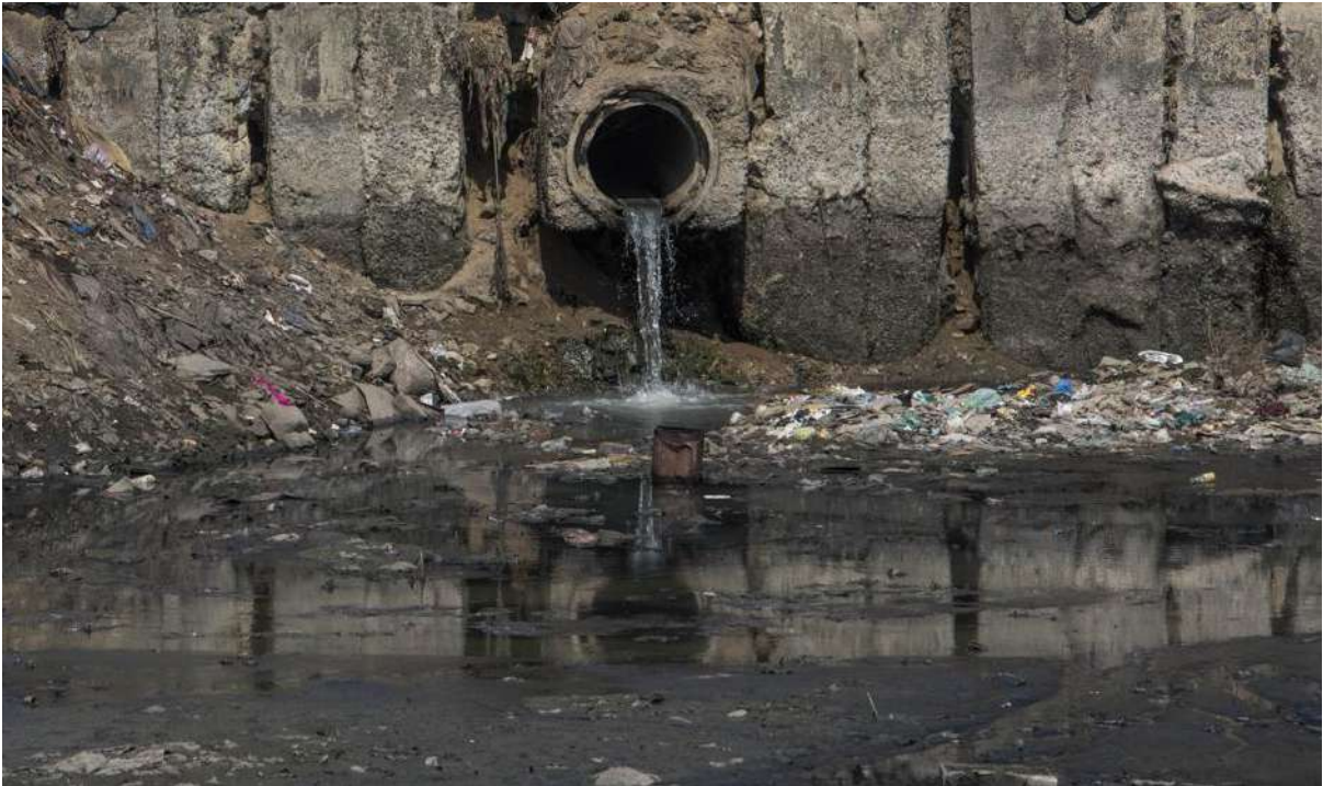
Waste water discharge points of factories near Raniganj
